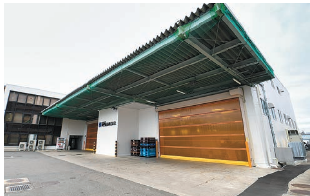
SLC (Shonai Logistics Center)
